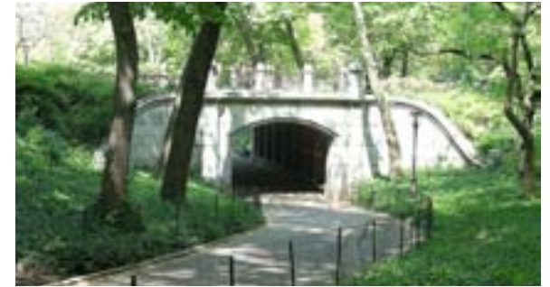
Figure 13. Pedestrian and bike underpass, Central Park, New York. Source: StephenRees, Flickr.
