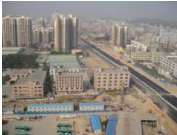
2. Aerial view of new arterial. Source: Kristin Simonson
