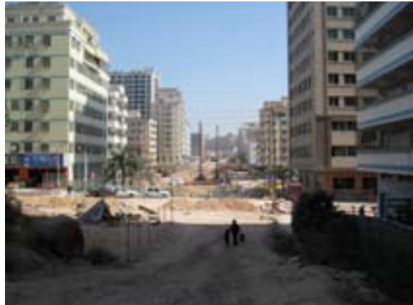
4. Boulevard under construction. Source: Kristin Simonson
