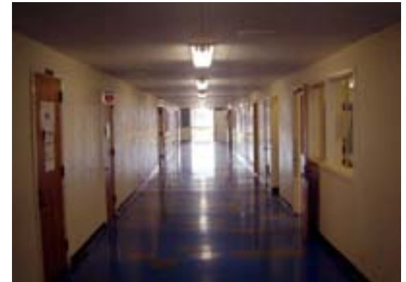
Halls of Carson High Source: www.hausmannconstruction.com
